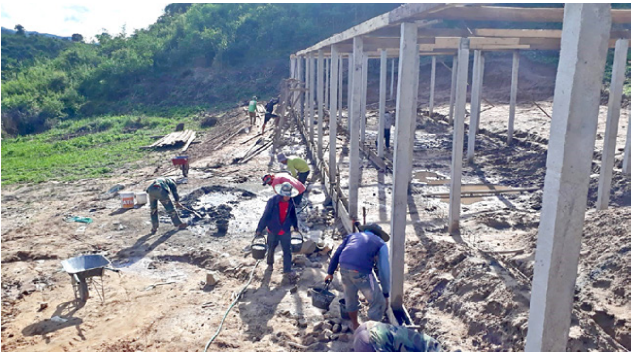
Villagers building a primary school in Oudomxay province, Lao P.D.R.
