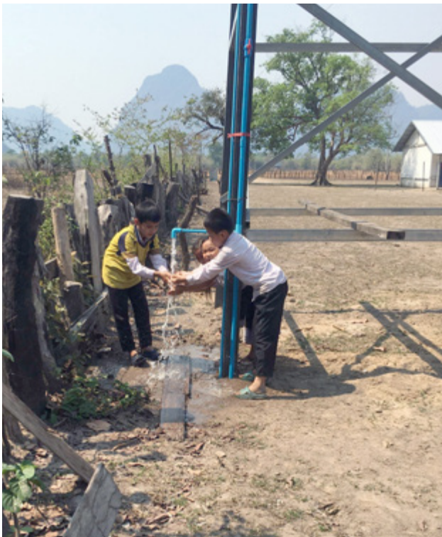
New water tower funded by A Child's Notebook and built by villagers for a primary school in Khammouane Province, Lao P.D.R.
