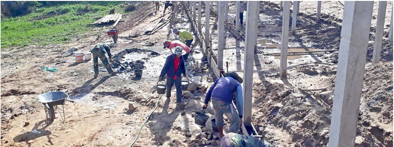
Villagers building a primary school in Oudomxay province, Lao P.D.R.
